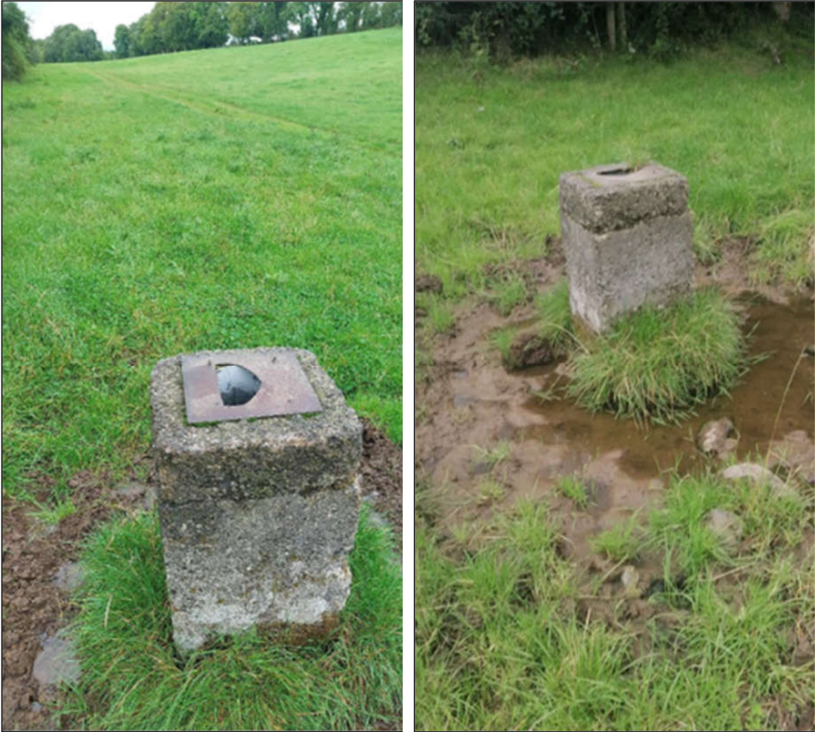
Plate 3 Existing well (condition unknown) (left: 2021, right: 2023)
