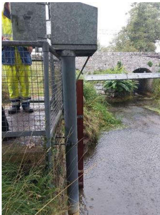
Figure 3: Aggard Bridge 29010 Hydrometric Station (facing downstream)
