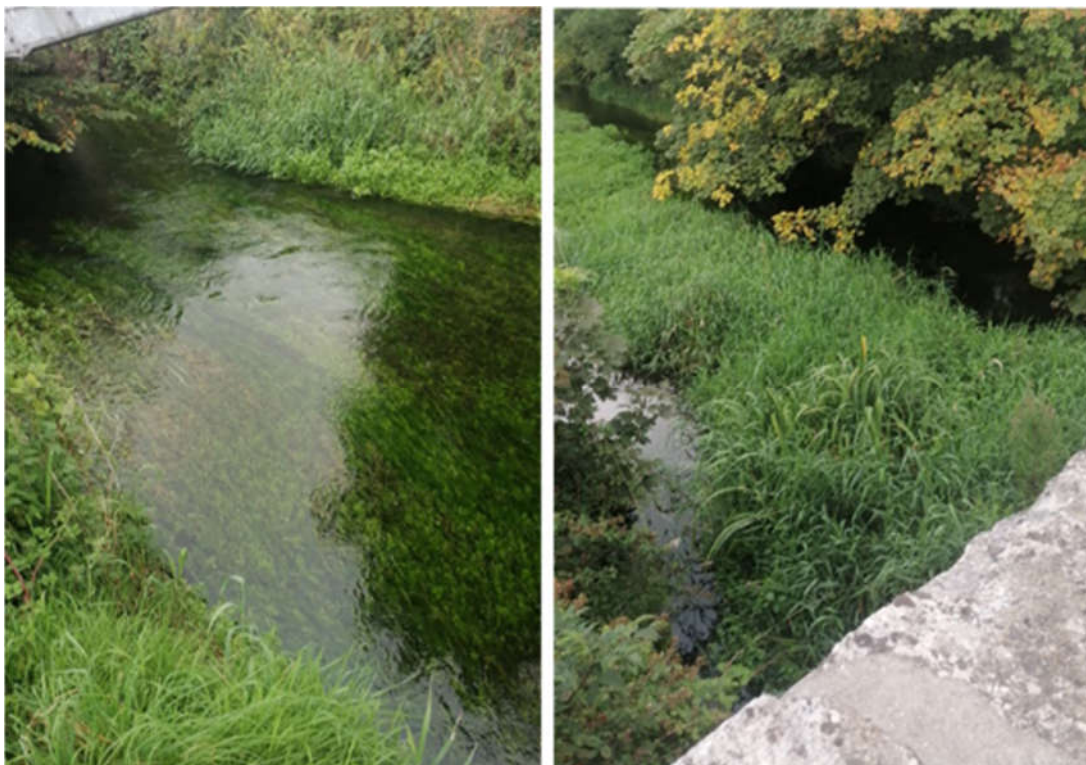
Figure 2: Overgrowth at Aggard Bridge
